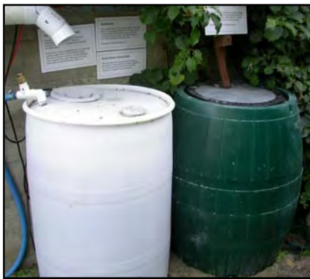
Panty hose (rear tank) and pool bag filters. Note: Vacuum breaker on white tank.
